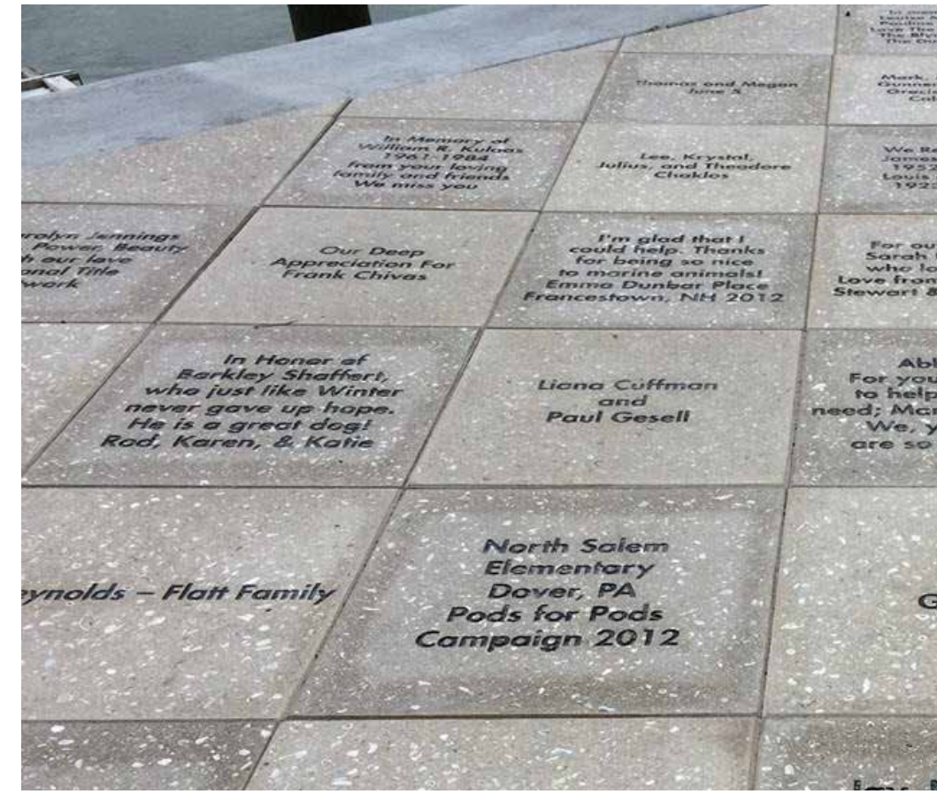
NEW PAVING W/MEMORIAL PAVERS
