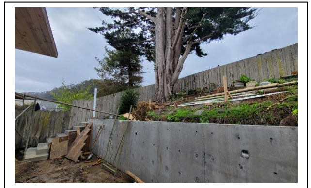
Compromised root plate. Root cutting at less than eight feet from the tree trunk.
