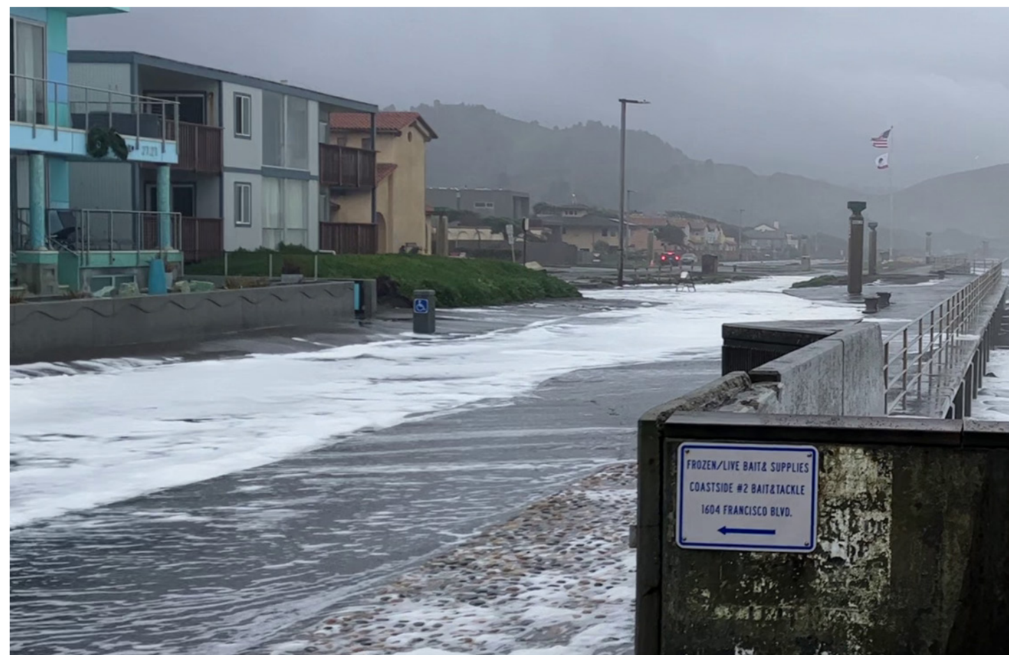
Storm flooding from wave overtopping along southern Beach Blvd
