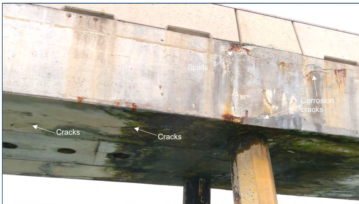
Figure A.3-44 Deck Exterior at Bent 1J - South Face
