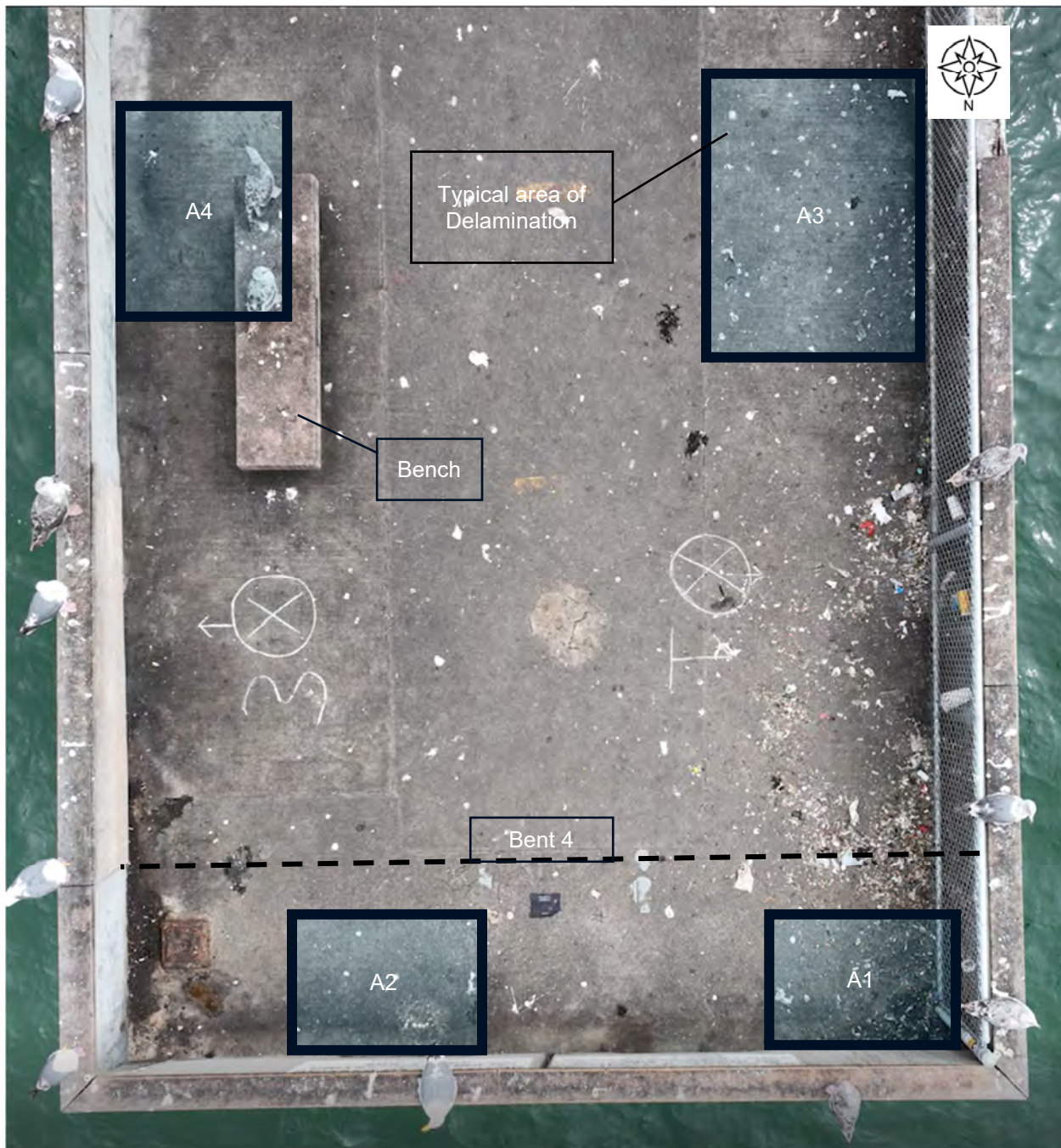
Figure A.2-1 Delaminated Areas at Bent 4 - N-S Extension Pier
