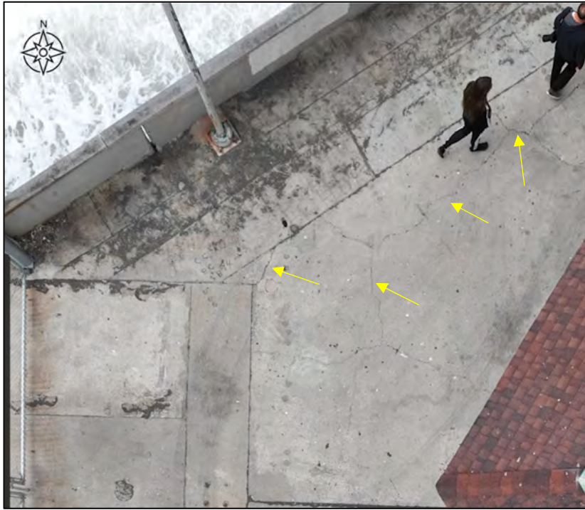
Figure 4.1 Visible Cracks on Abutment 1-A - Main Pier Entrance
