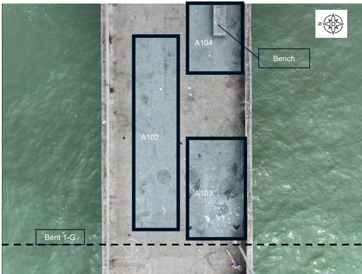
Figure A.2-34 Delaminated Areas around Bent 1-G – E-W Main Pier
