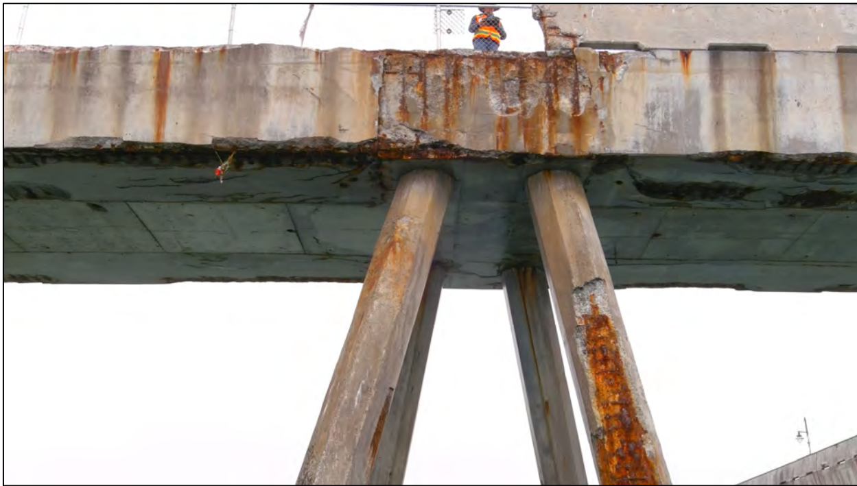
Figure 4.10 Bent Severe Rating (Bent 3)
