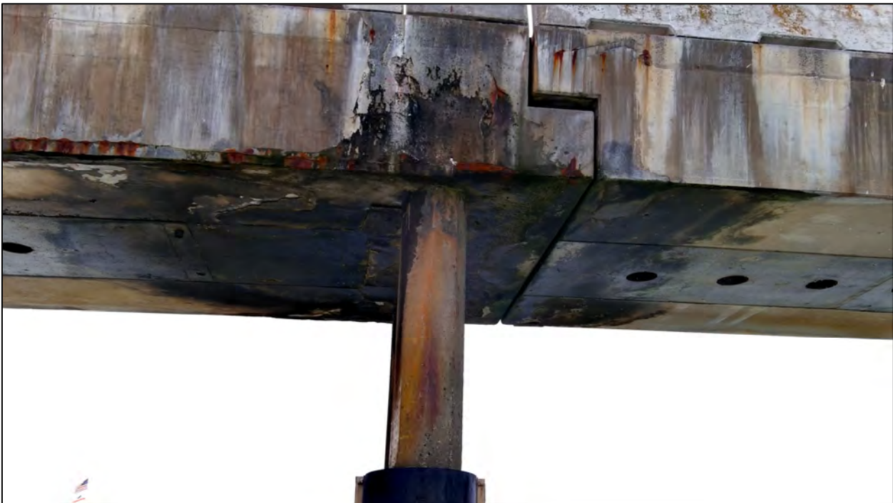
Figure 4.9 Bent Major Rating (Bent 1B)
