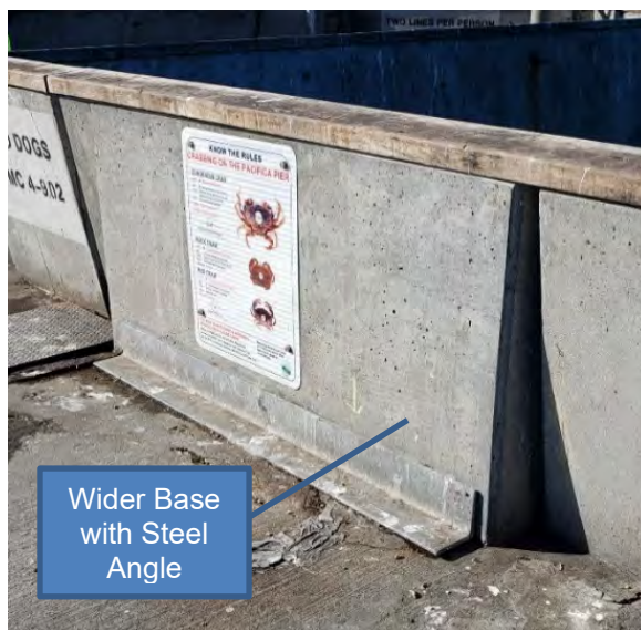
Figure 10: Repaired Handrail Panel
