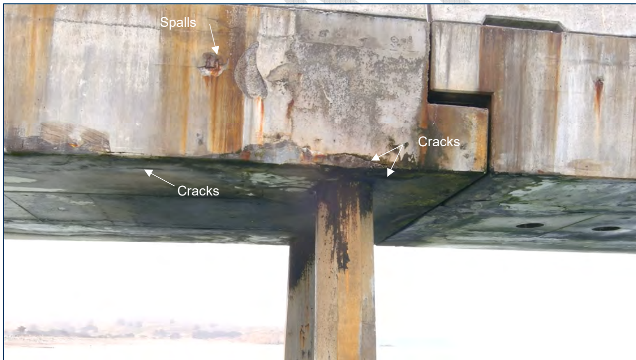
Figure A.3-35 Deck Exterior at Bent 1H – North Face
