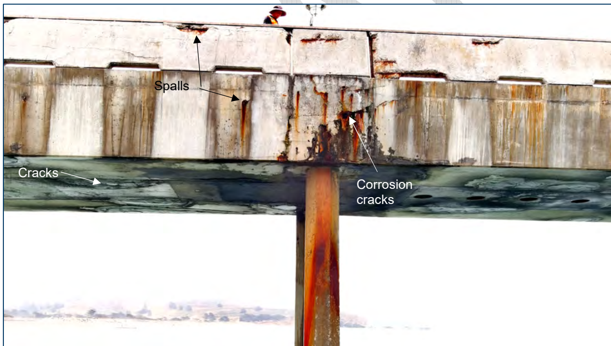
Figure A.3-32 Deck Exterior at Bent 1G – North Face
