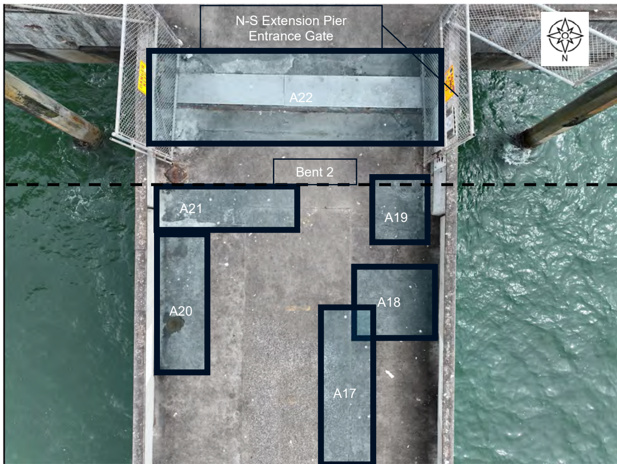
Figure A.2-7 Delaminated Areas at Bent 2 - N-S Extension Pier Entrance
