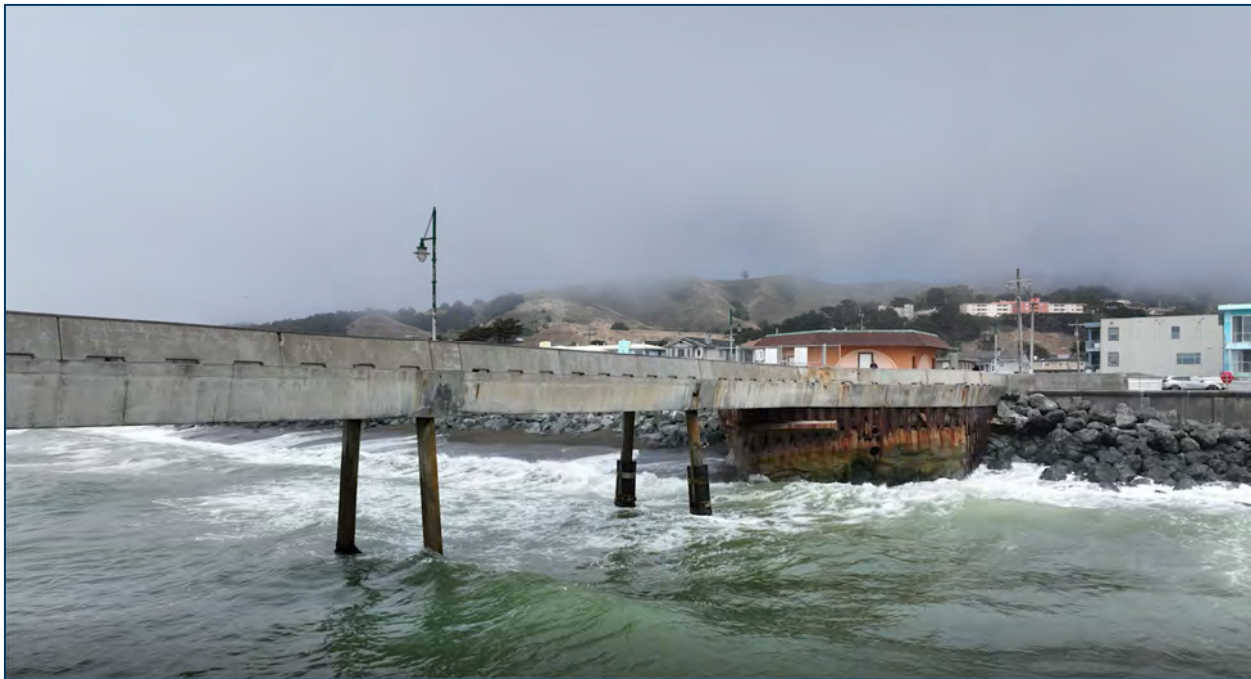
Figure A.3-12 Deck Exterior between Bent 1C and Pier Abutment – South Face
