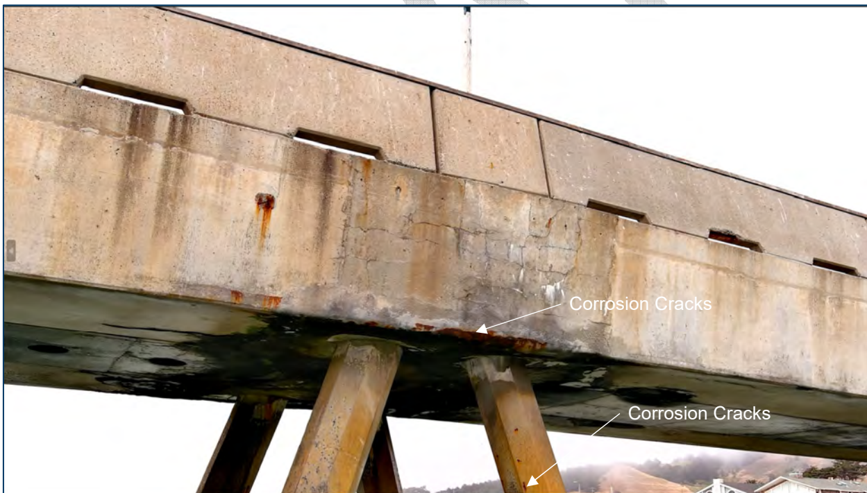
Figure A.3-25 Deck Exterior at Bent 1E – South Face
