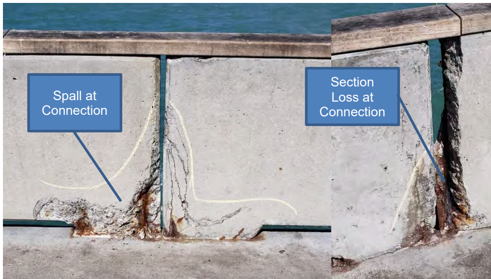
Figure 8: Typical Damage Rated Severe
