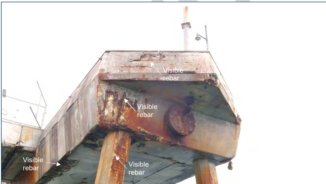
Figure A.3-74 Deck Exterior at Bent 1R and N-S Pier Extension Joint – North - West Face
