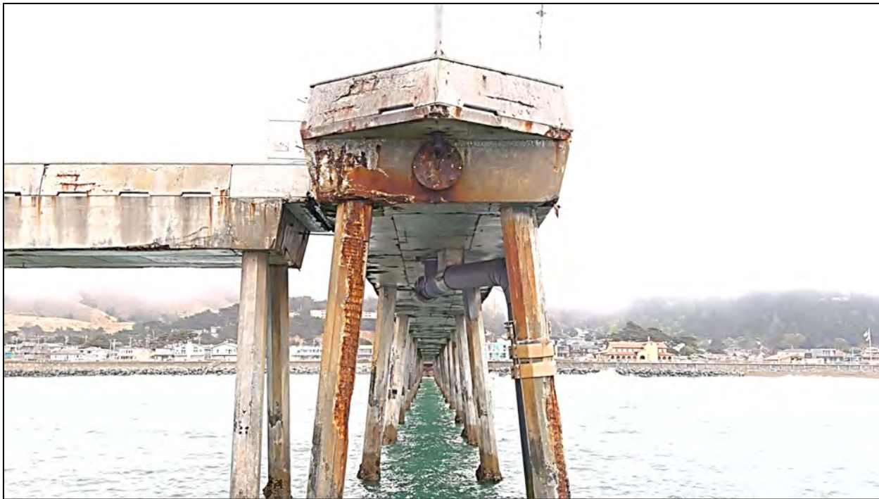
Figure 4.16 Pile Damage Rating - Severe (Bent 1R)
