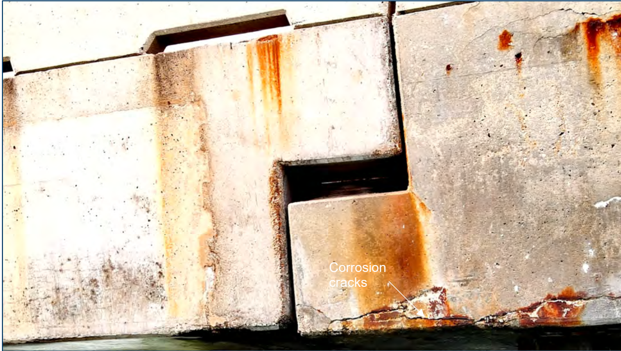
Figure A.3-90 Bearing Plate at Deck and Bent Connection
