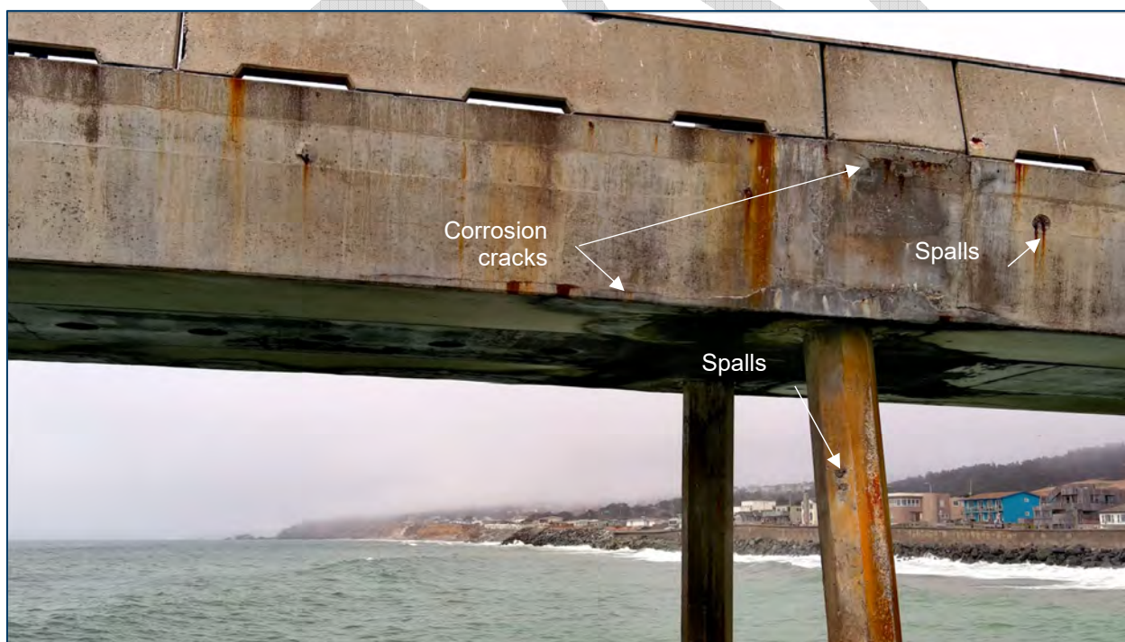
Figure A.3-29 Deck Exterior at Bent 1F – South Face
