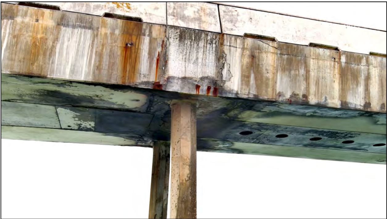
Figure 4.7 Deck Major Rating (Bent 1F)
