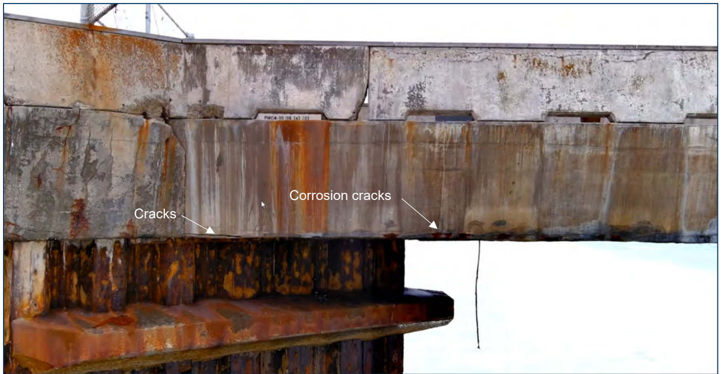
Figure A.3-7 Deck Exterior between Pier Abutment and Bent 1B – North Face
