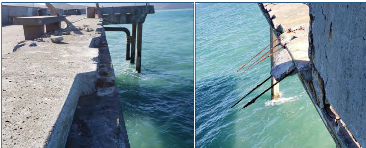
Figure 3.1 Collapsed Handrail, Photo 2021
