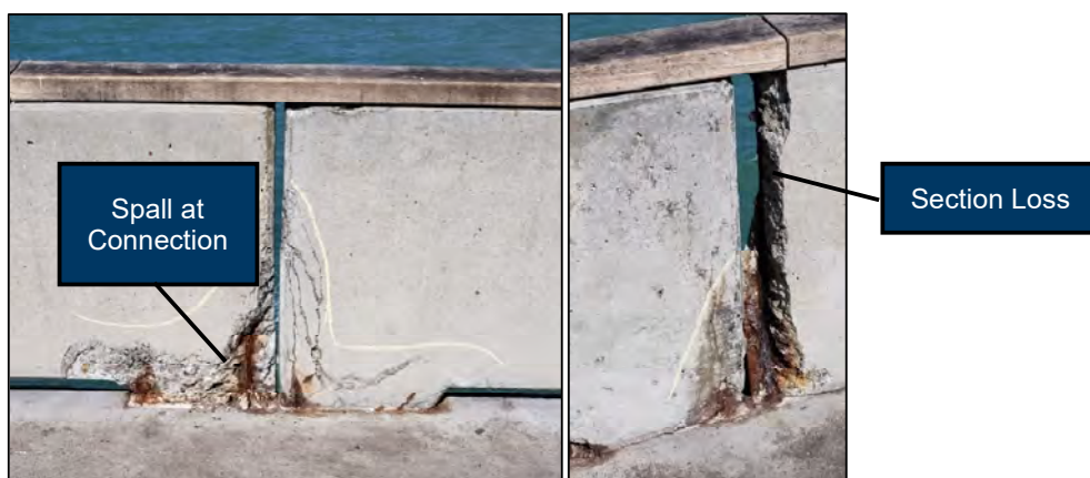
Figure 3.5: Typical Damage Rated Severe
