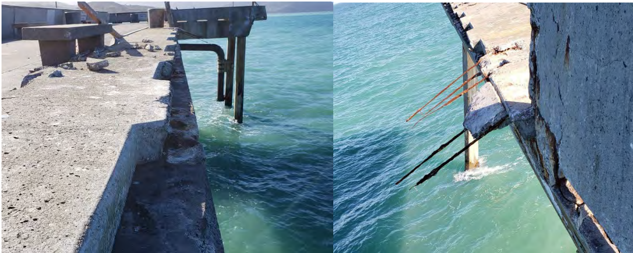
Figure 4: Photos of Collapsed Handrail
