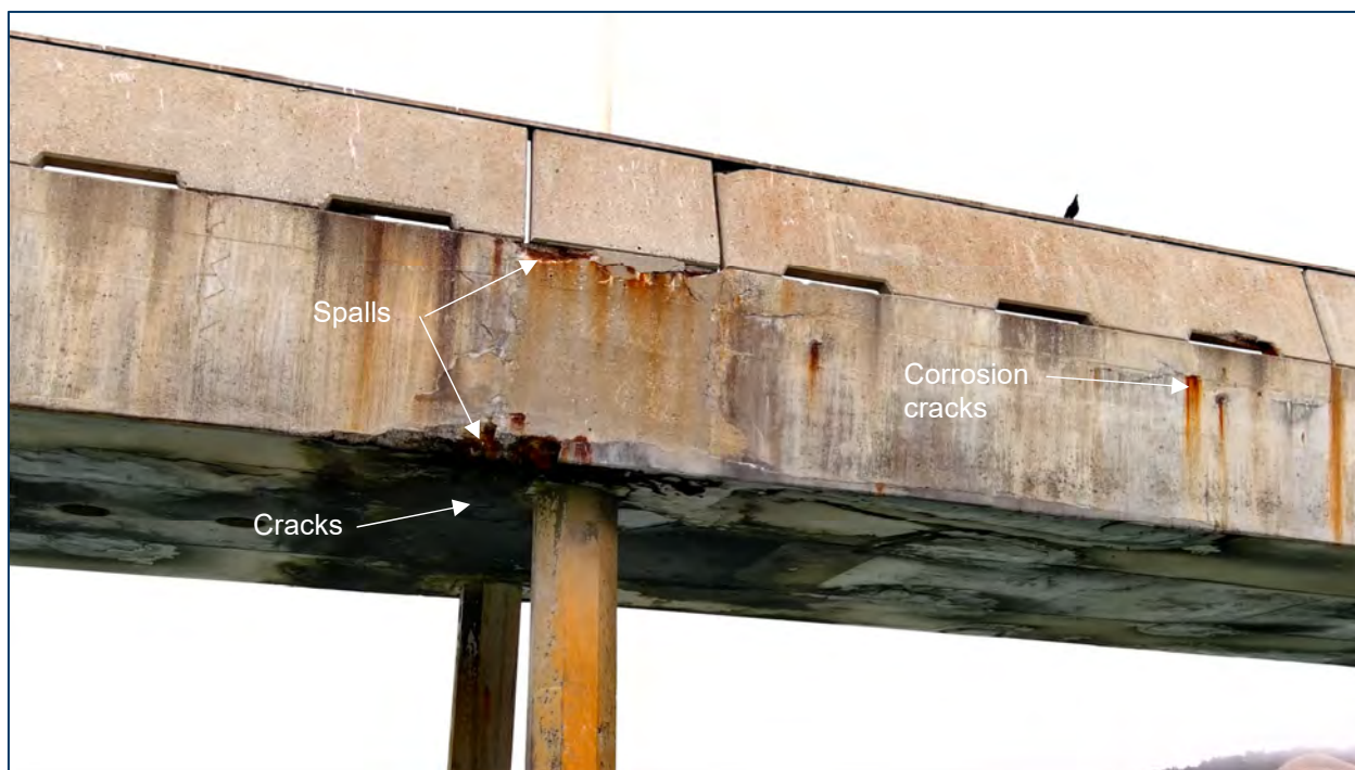
Figure A.3-33 Deck Exterior at Bent 1G – South Face
