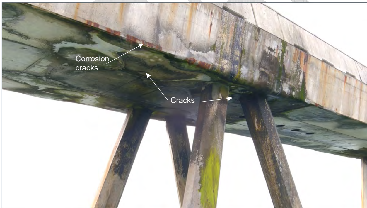
Figure A.3-46 Deck Exterior at Bent 1K – North Face
