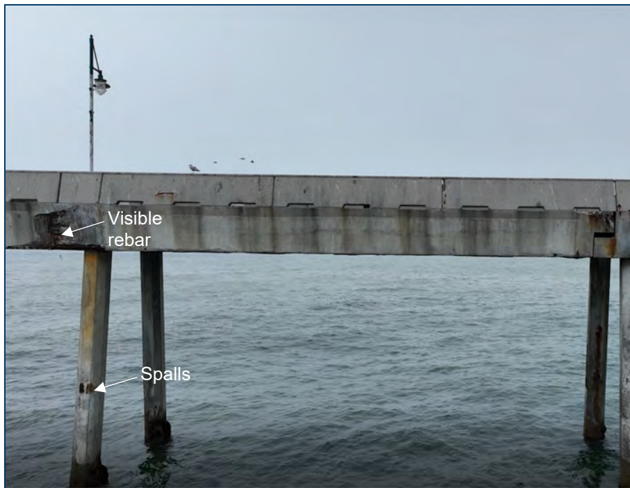
Figure A.3-59 Deck Exterior between Bent 10 and 1N – South Face
