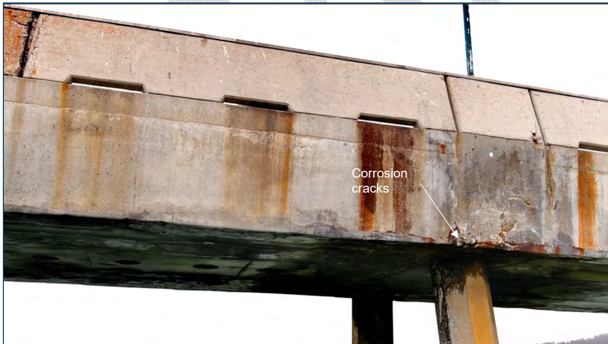
Figure A.3-40 Deck Exterior at Bent 1I – South Face
