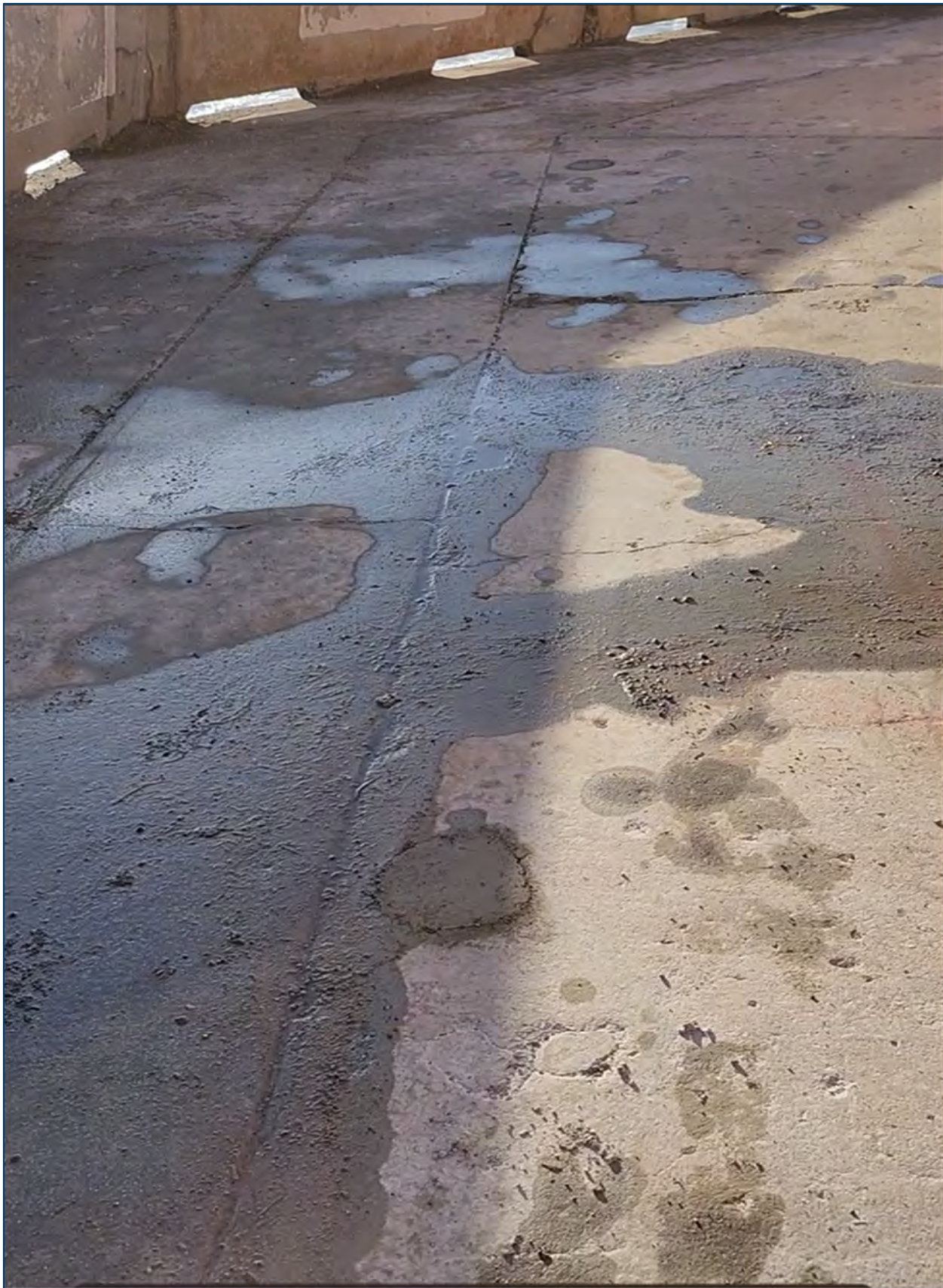
Figure A.1-24 Typical photo of hole filled after drilling
