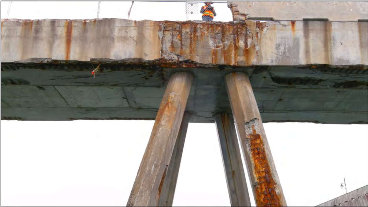
Figure 4.8 Deck Severe Rating (Bent 3)
