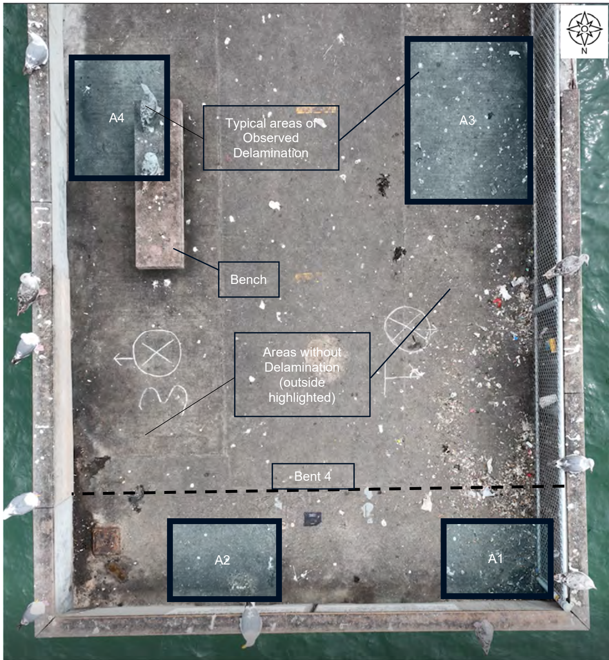
Figure 4.5 Delaminated Areas at Bent 4 - N-S Extension Pier
