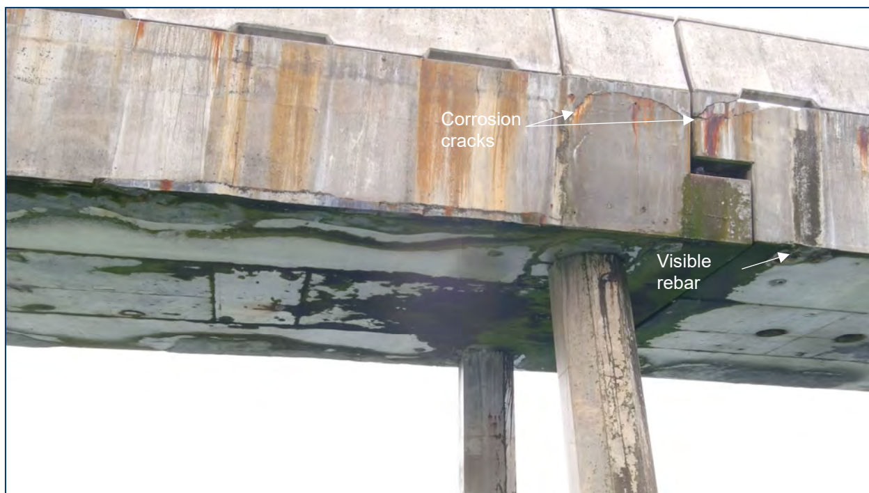
Figure A.3-56 Deck Exterior at Bent 1N – North Face
