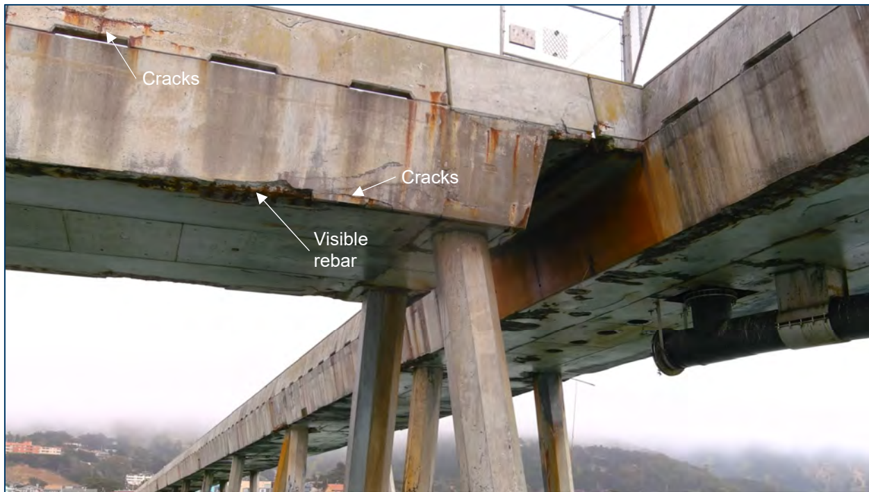
Figure A.3-80 Deck Exterior at Bent 2 and N-S Pier Extension Joint – West Face
