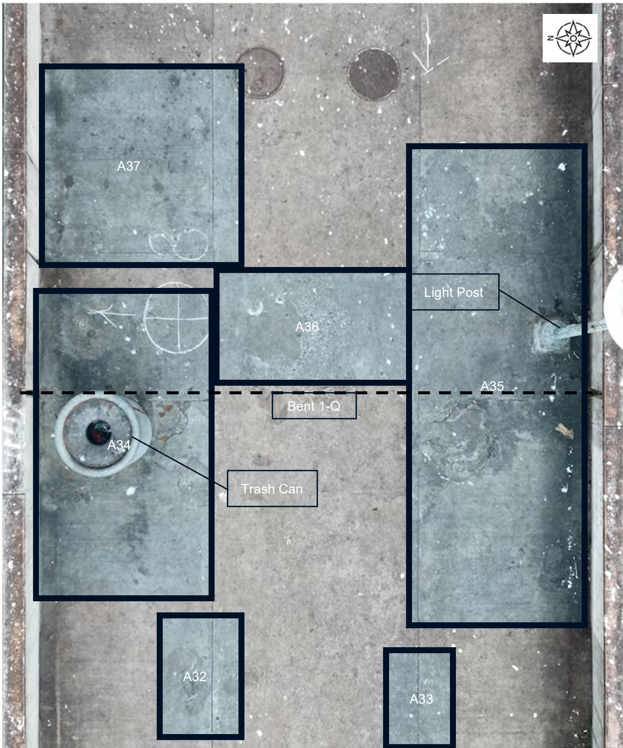
Figure A.2-10 Delaminated Areas at Bent 1-Q - E-W Main Pier
