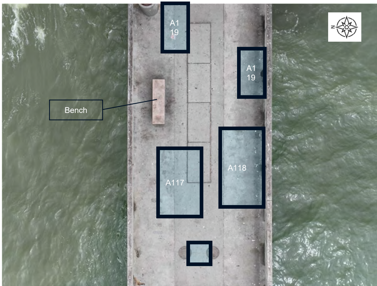
Figure A.2-39 Delaminated Areas between Bent 1-C and Bent 1-D – E-W Main Pier
