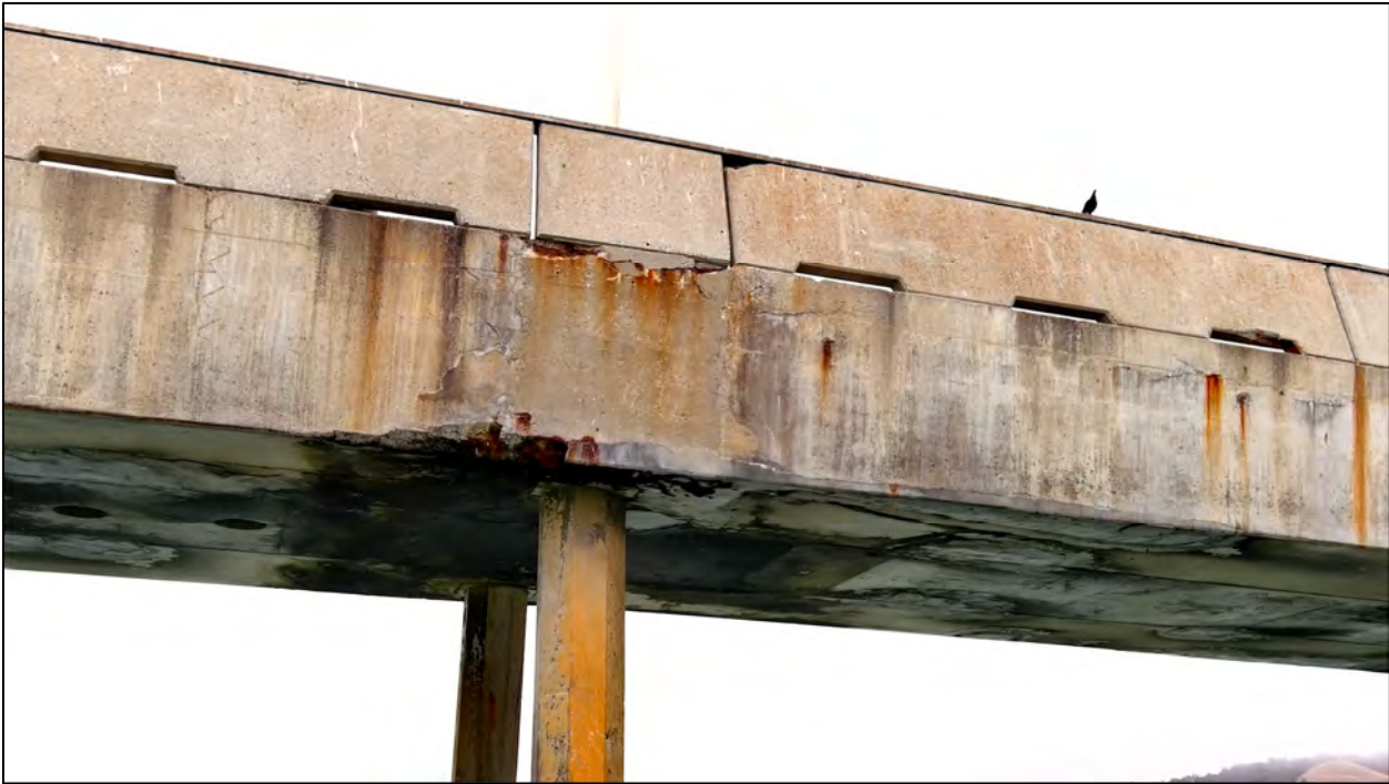
Figure 4.14 Pile Damage Rating - Moderate (Bent 1G)
