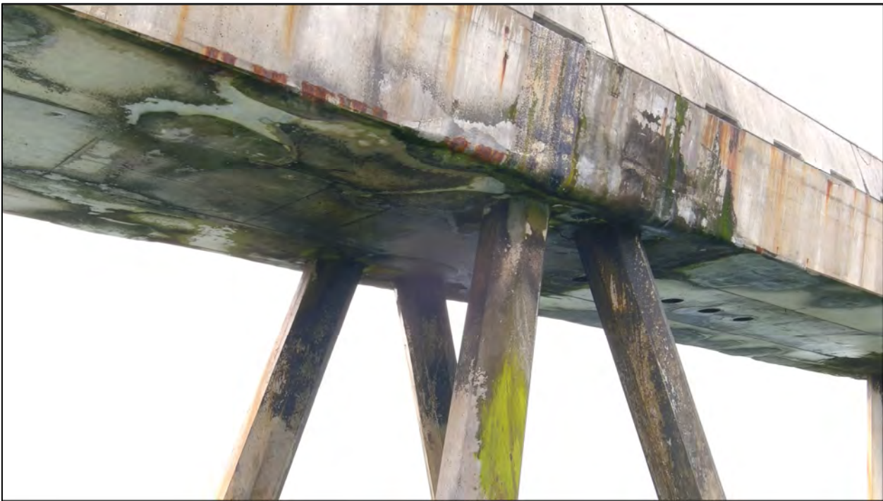
Figure 4.15 Pile Damage Rating - Major (Bent 1K)
