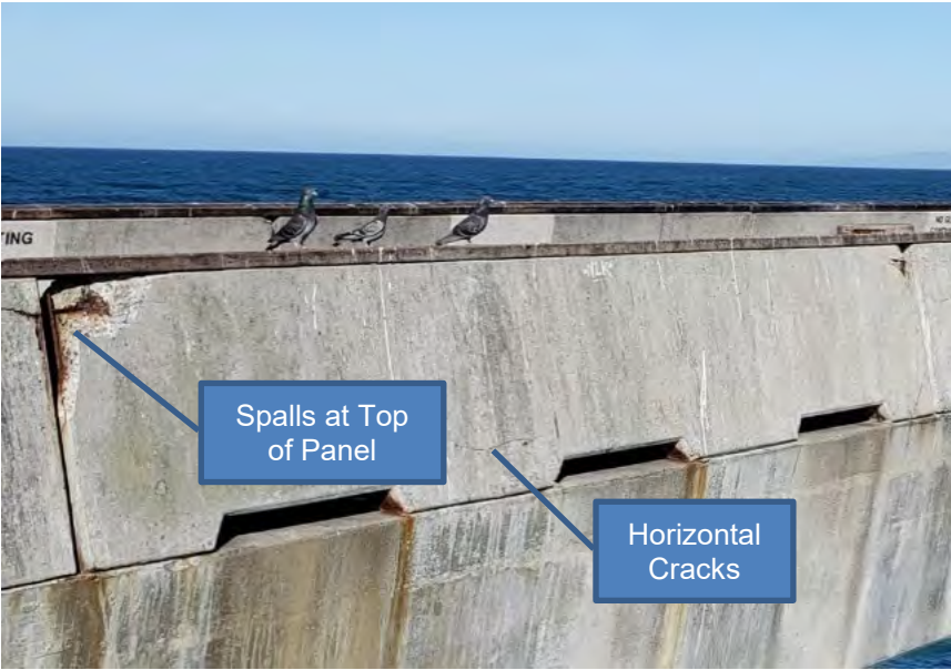
Figure 6: Typical Damage Rated Moderate
