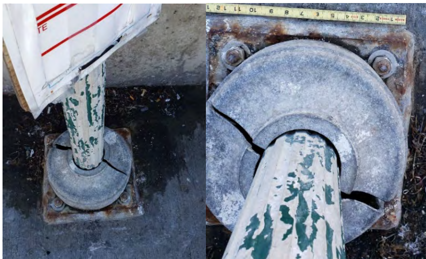
Figure 9: Typical Light Post Foundation
