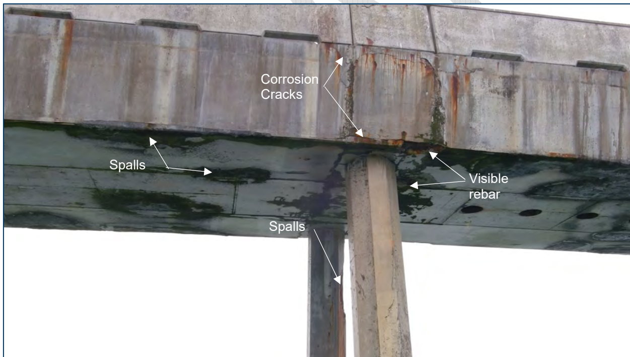
Figure A.3-60 Deck Exterior at Bent 10 - North Face
