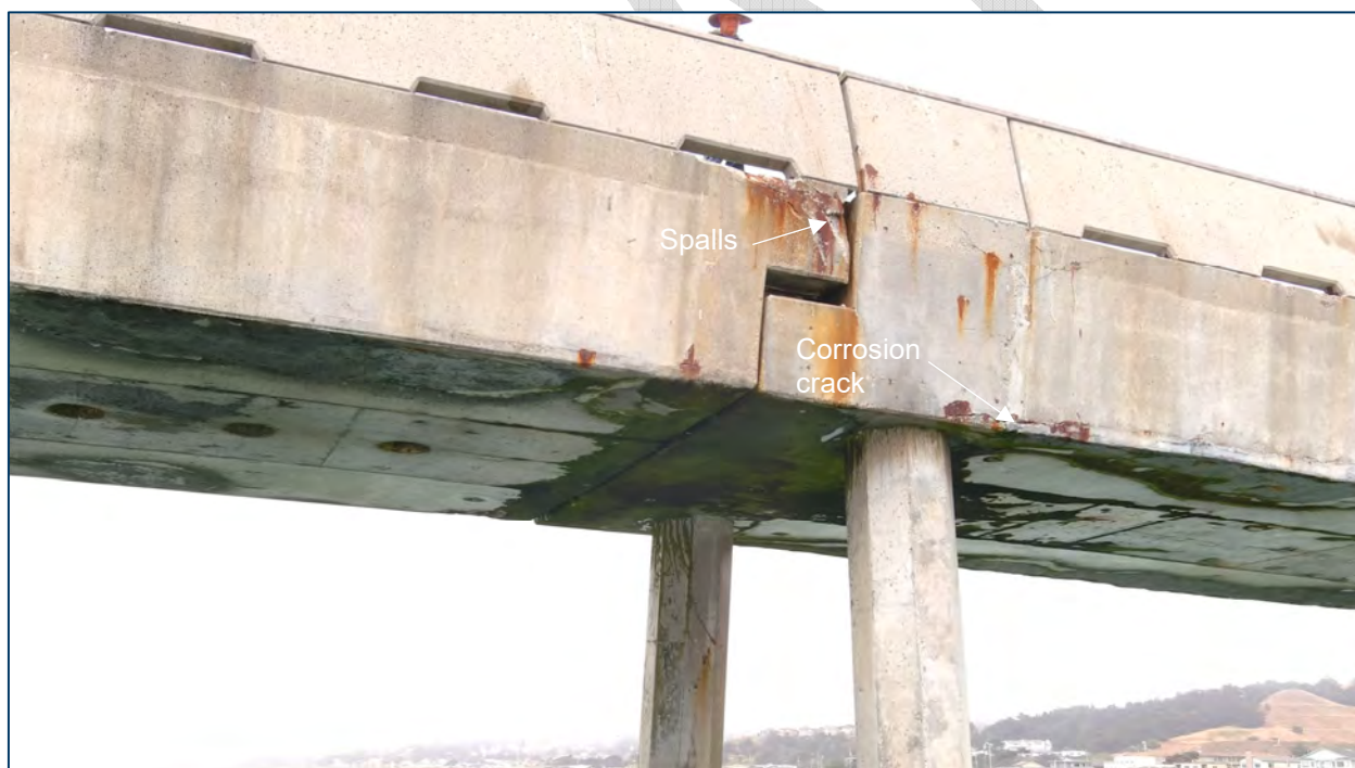
Figure A.3-57 Deck Exterior at Bent 1N - South Face
