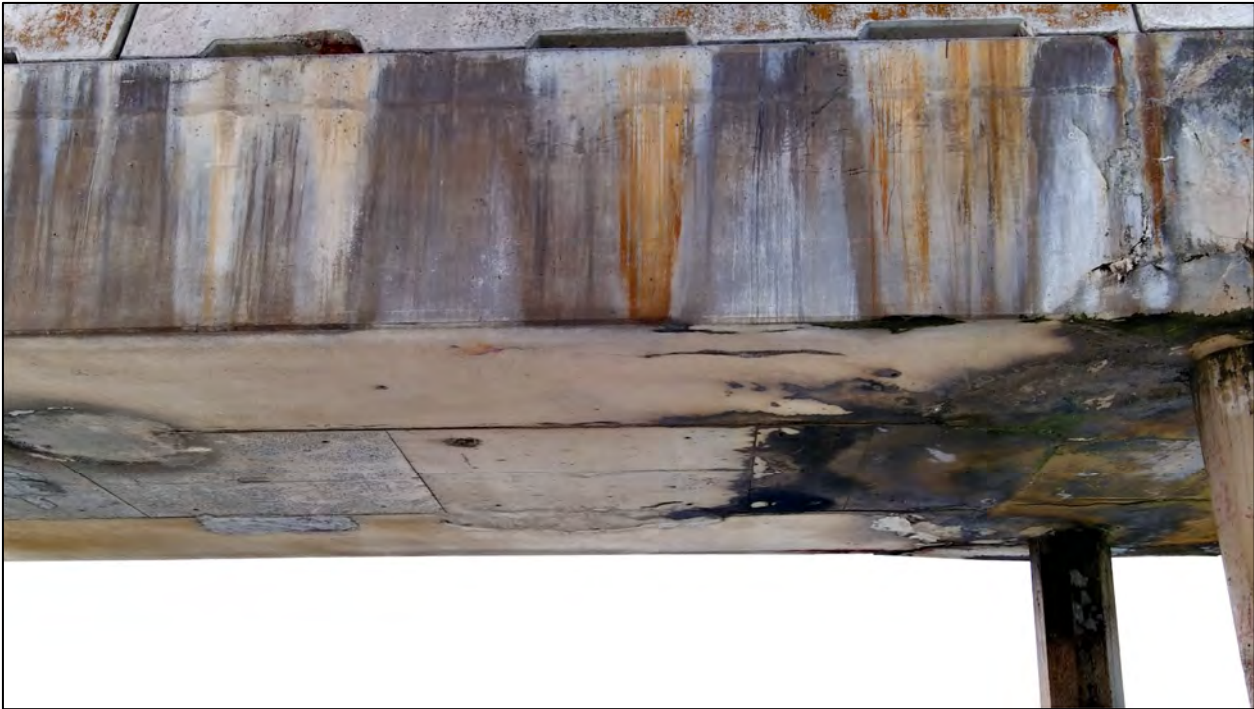
Figure 4.6 Deck Moderate Rating (Bent 1C)
