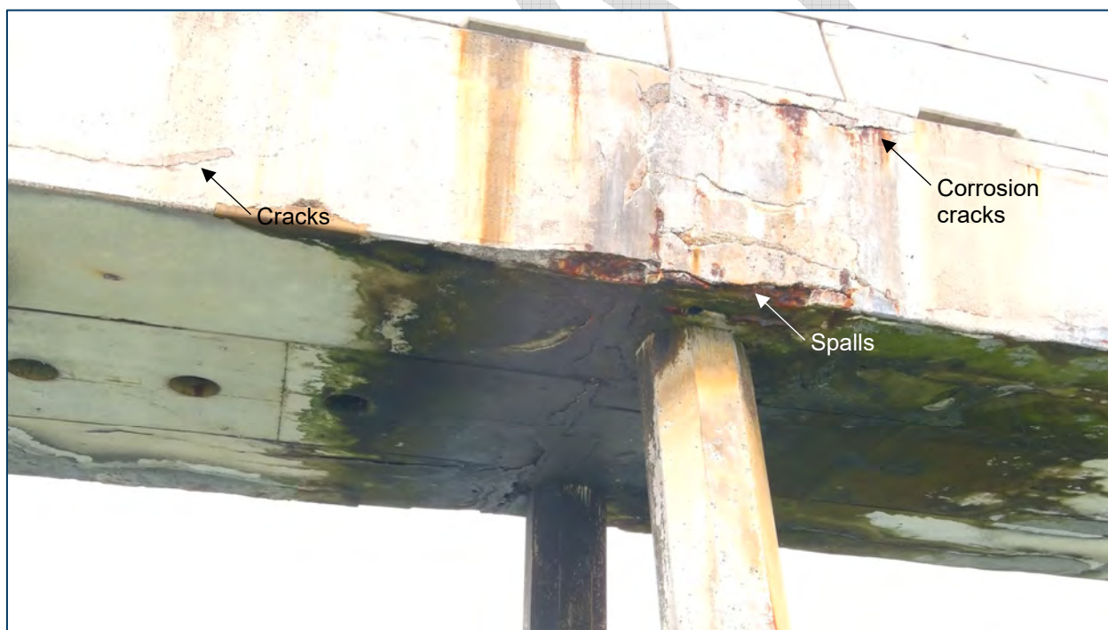
Figure A.3-50 Deck Exterior at Bent 1L – South Face
