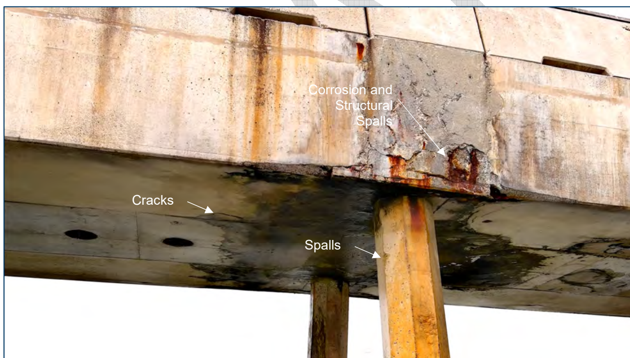
Figure A.3-20 Deck Exterior at Bent 1D – South Face
