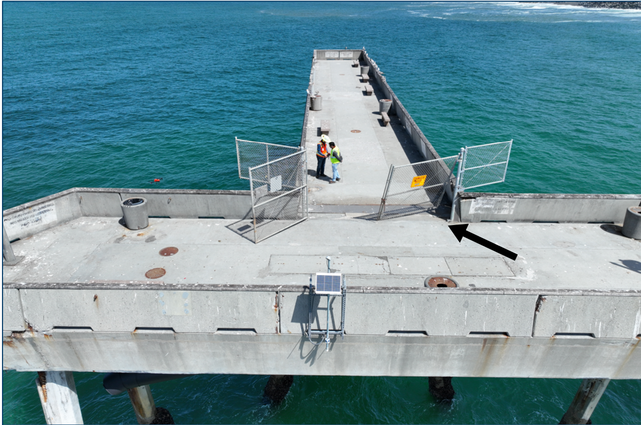
Figure 3.12 Chain-link Fence between Main Pier and Pier Extension
