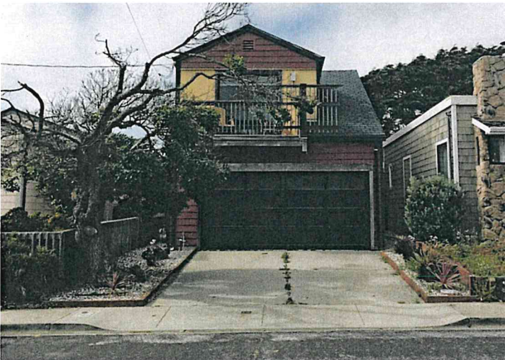
San Jose Avenue: Frontage dominated by garage, limited front yard landscaping, entry on side, on-street parking unavailable, driveway parking available.
