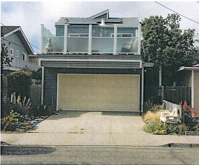
Salada Avenue: Frontage dominated by garage, limited front yard landscaping, entry on side, on-street parking unavailable, driveway parking available.
