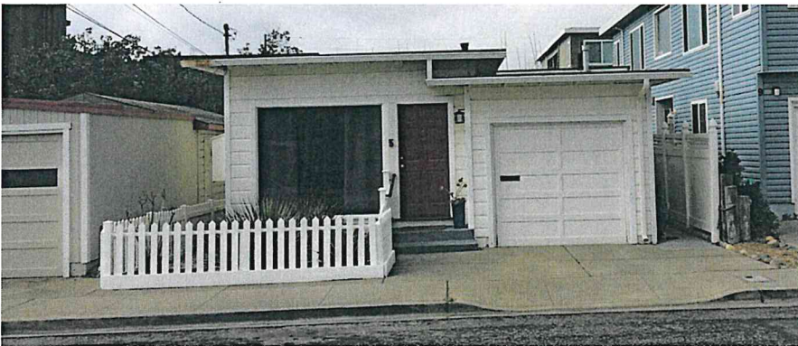
Salada Avenue: Frontage dominated by one-car garage, moderate front yard landscaping, entry on front, on-street parking available, driveway parking unavailable.
