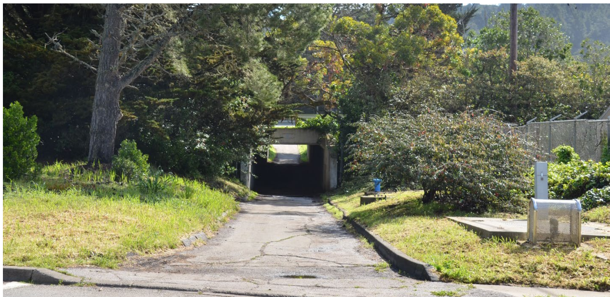
The Highway 1 Tunnel, looking east from Bradford Way.
