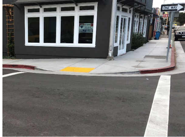
A curb ramp for the Carmel Avenue crossing at Francisco Boulevard.
