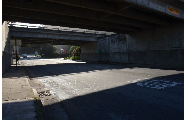
The Clarendon Road underpass.
