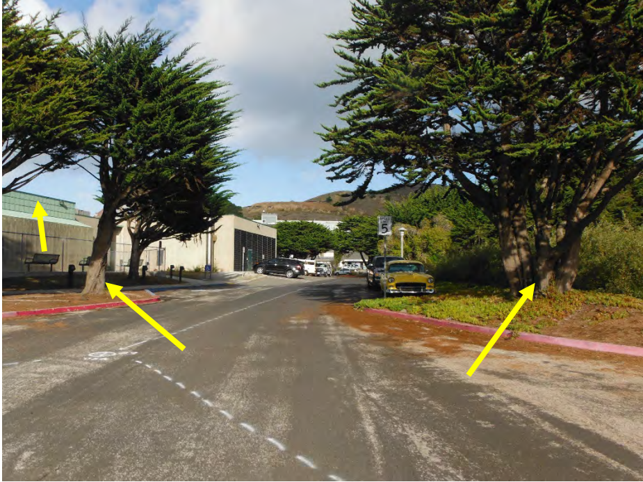
Photograph 1: Facing northeast, the asphalt-covered driveway and Pacifica Community Center (left). Yellow arrows indicate trees to be removed during construction process.
