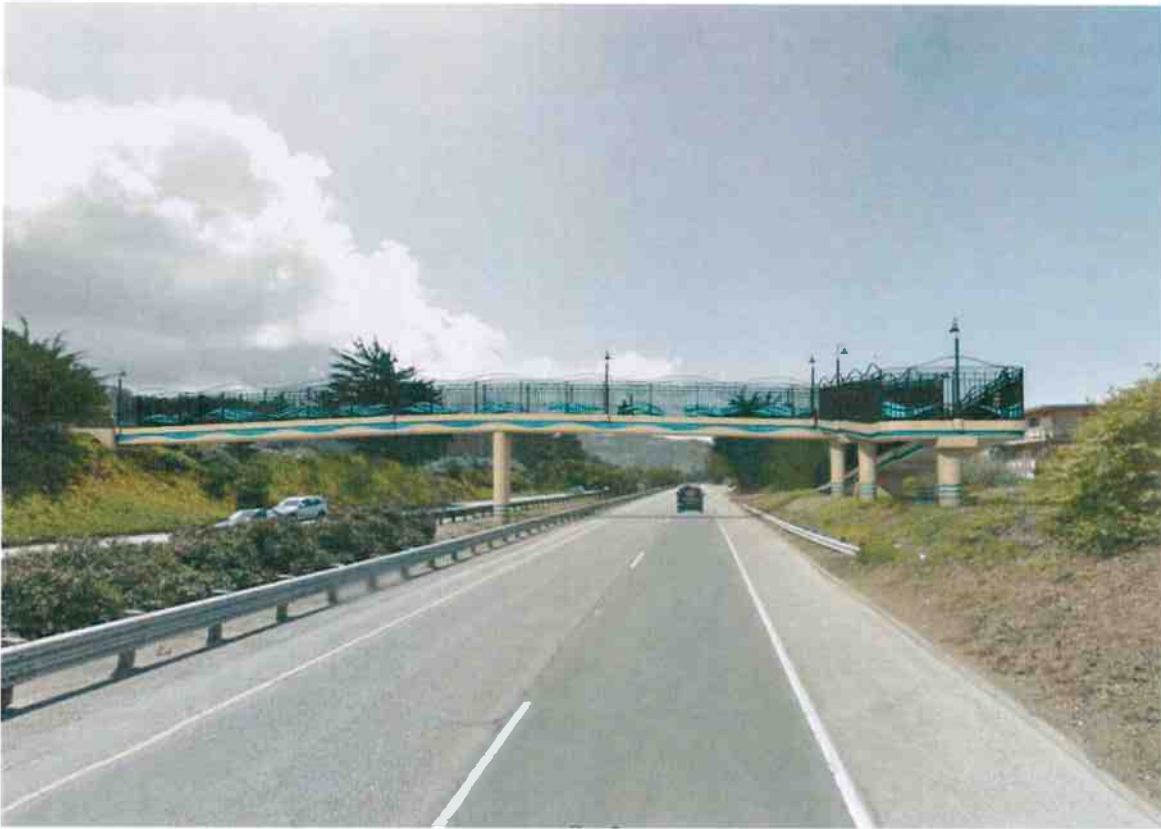
San Jose Ave POC (Replace) looking south
