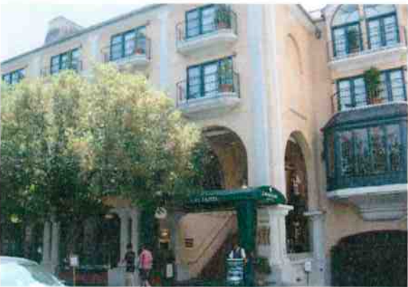
New development in Mixed Use Neighborhood areas should include multi-family housing or ground-floor commercial uses with housing above (top). The Mixed Use Center classification is intended for high-density mixed use development, hotels, or community uses (middle). The Visitor-Serving Commercial classification promotes concentrated development of commercial uses with visitor appeal (bottom).
