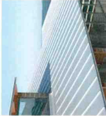
LIGHT STANDING SEAM ROOF 5
