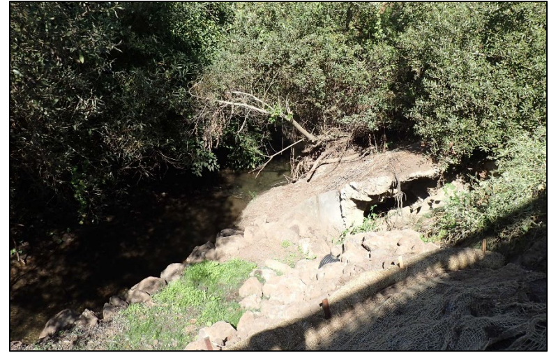
View looking down at storm drain outfall towards San Pedro Creek.
