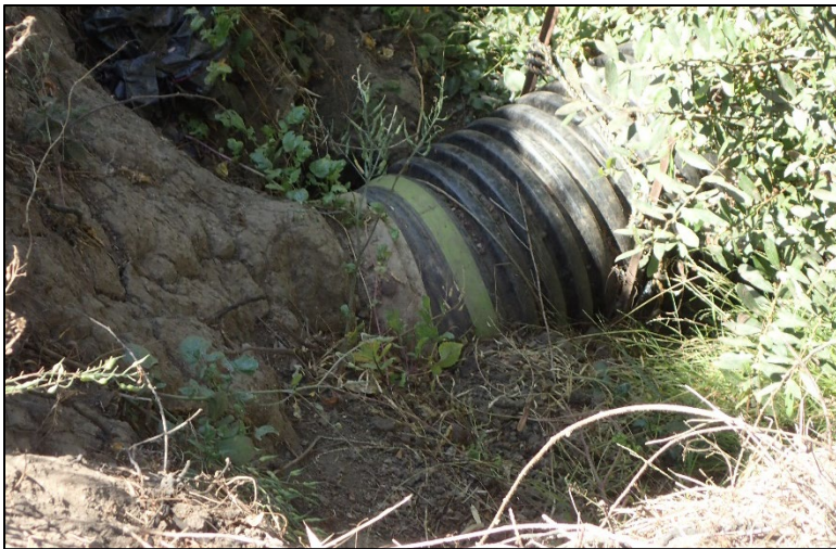
View of existing storm drain.
