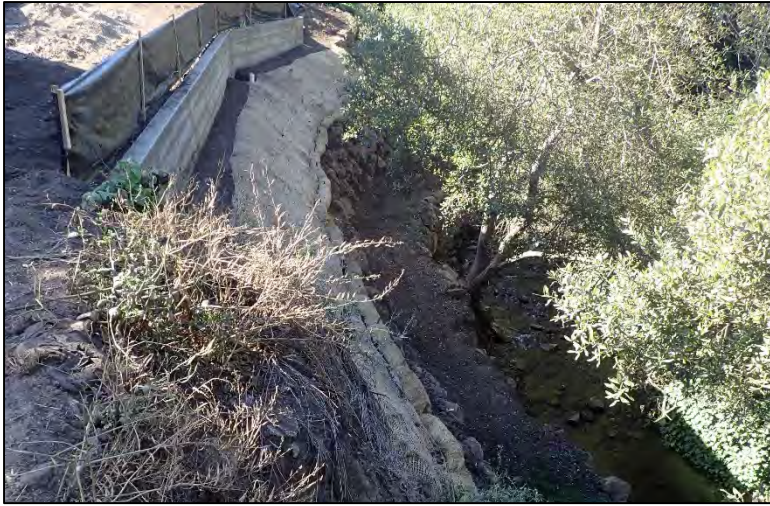
Photograph 1. View of bank stabilization adjacent to the project area. Photo taken from the north bank facing upstream from culvert (09/20/2019).
