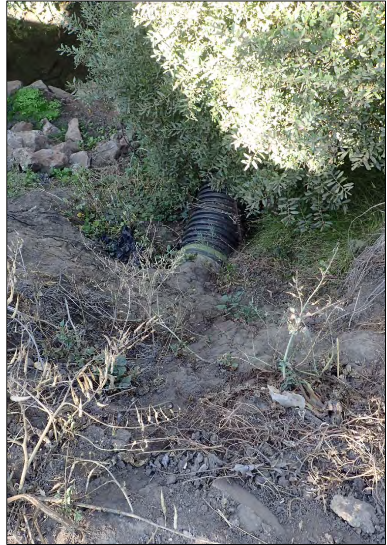
Photograph 5. View of the existing outfall structure from above (taken 09/20/2019).
