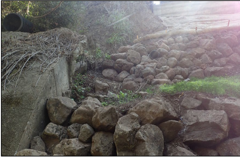
View of existing storm drain outfall and riprap.
