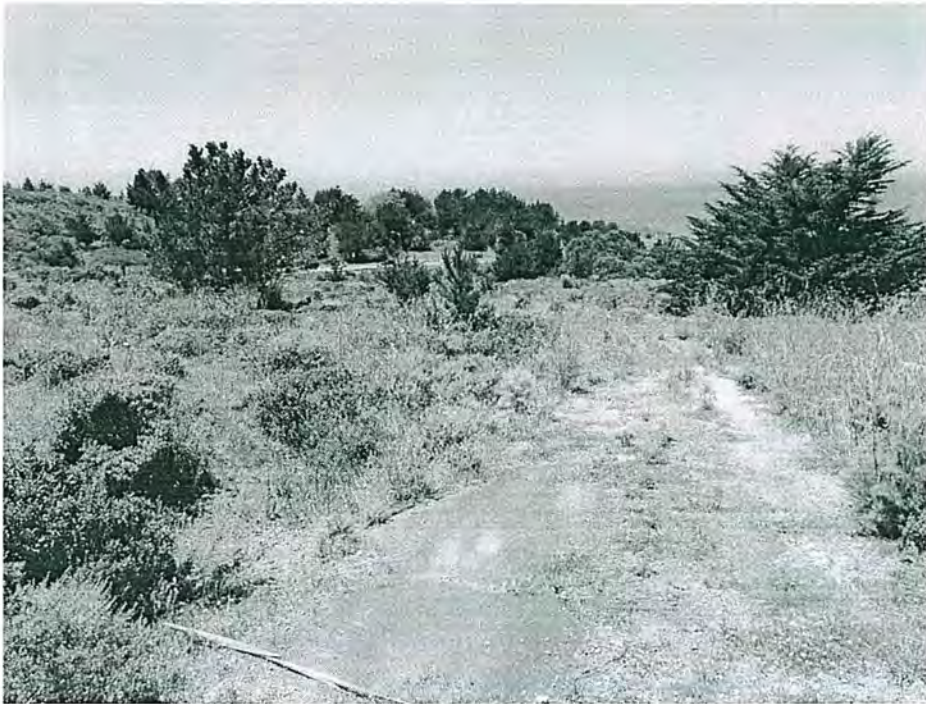
Photo 3. Existing asphalt road that will be restored.
