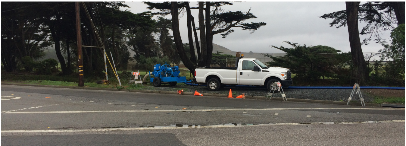
Figure 16 Portable stormwater pump station at Clarendon Road and Lakeside Avenue (1/9/2018)
