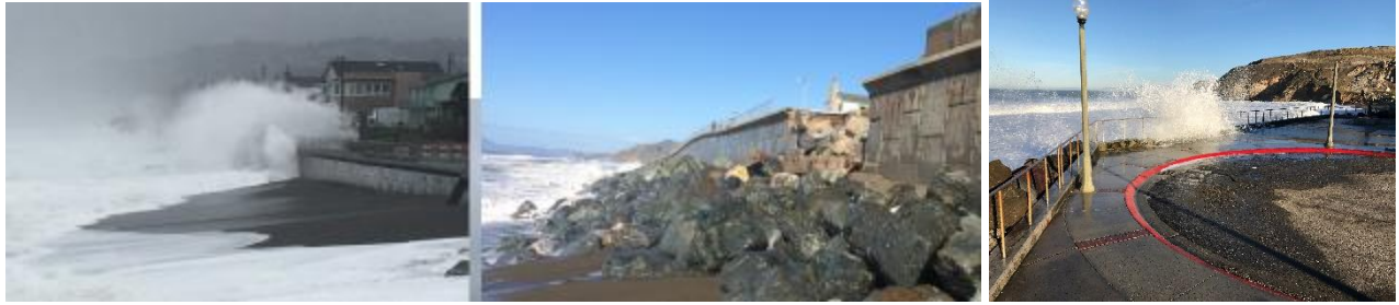
Figure 2 Wave overtopping at Beach Blvd (left) on January 22, 2016 and seawall damage (center); Rockaway on November 30, 2017 (right)
