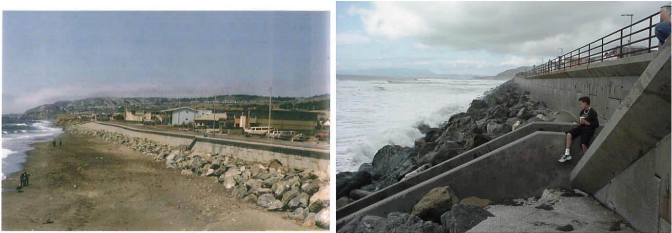
Figure 6 Beach Blvd seawall in 1985 (left) after construction and in 2010 (right) showing no beach at high tide.
