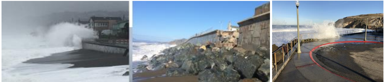
Figure 2 Wave overtopping at Beach Blvd (left) on January 22, 2016 and seawall damage (center); Rockaway on November 30, 2017 (right)
