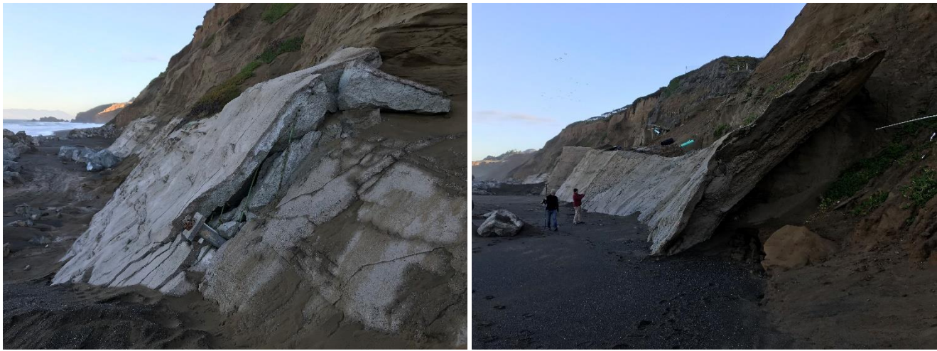
Figure 3 Structural failure of Land’s End Seawall (left) and erosion beyond end (right)
