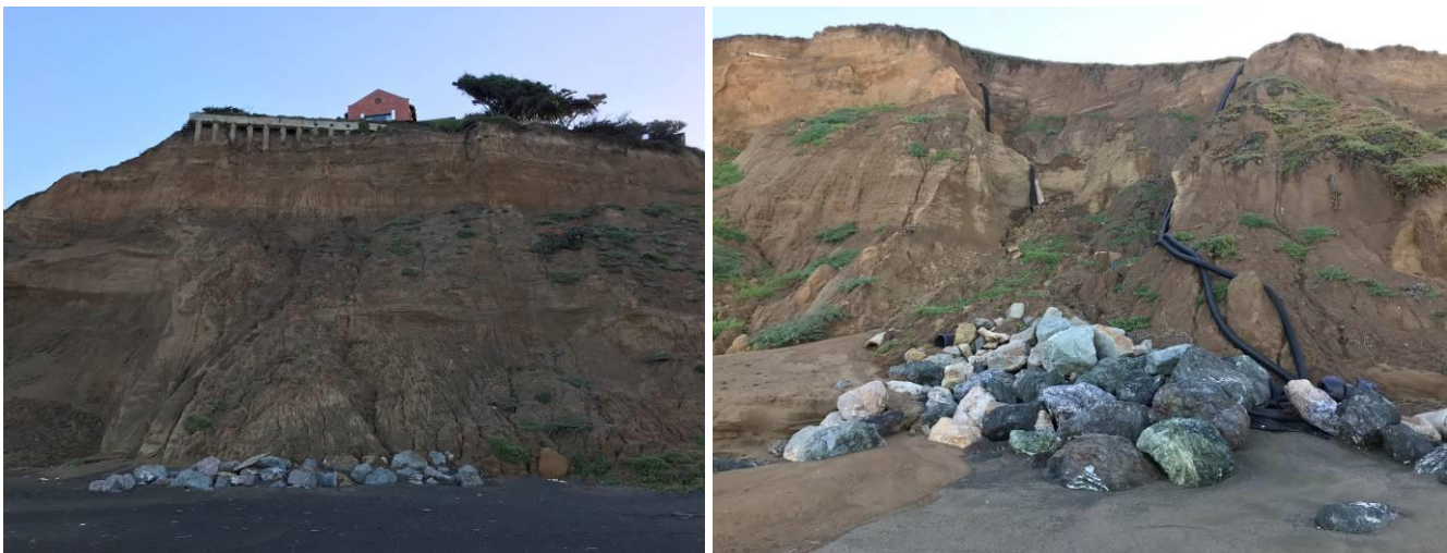
Figure 6 Dollaradio Station with rock at toe and Piles at top of bluff (Left) Drainage pipes and terrestrial erosion of bluff south of Dollar Radio (Right)
