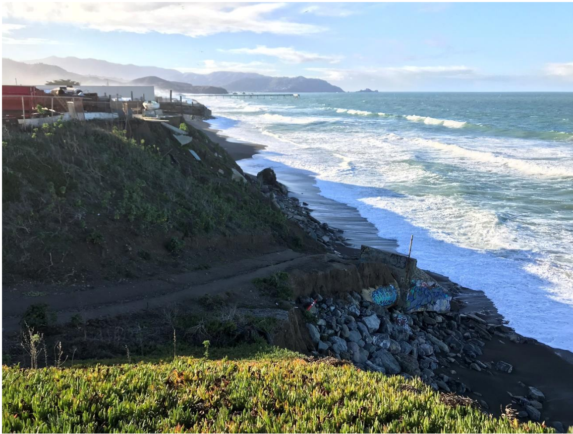
Figure 13 Damaged stormwater outfall in foreground, landfill and eroded rubble on narrow beach beyond
